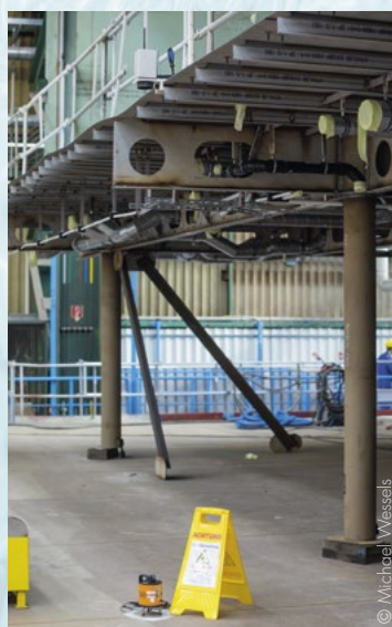
In the construction dock (left), self-levelling lasers (centre) and precision detectors (right) ensure millimetre-precise positioning of the sections weighing several tons.
